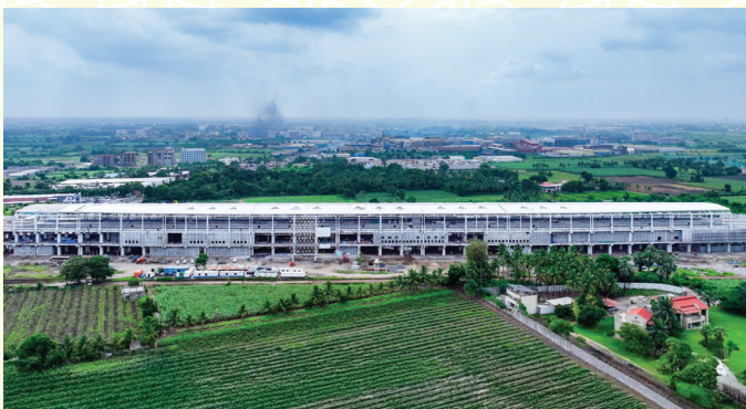
Under Construction Surat Bullet Train Station
